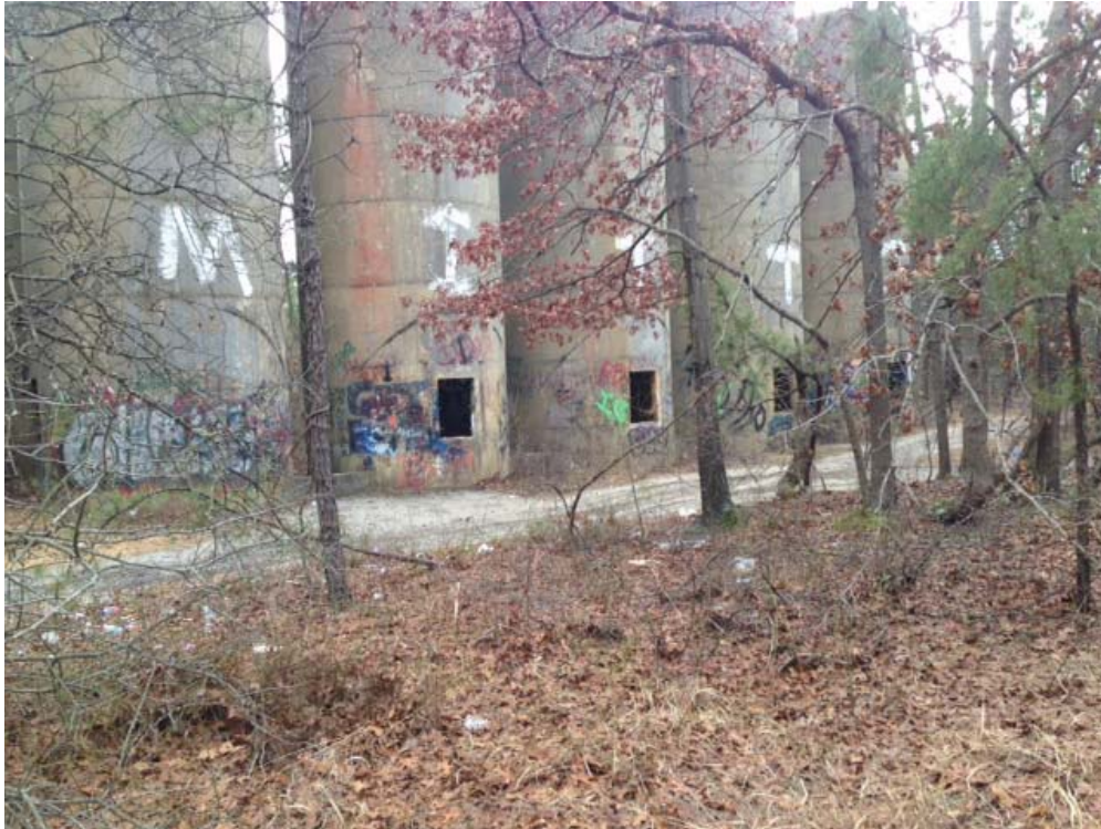
5. Abandoned silos located within the northern portion of the survey area along northern property boundary
